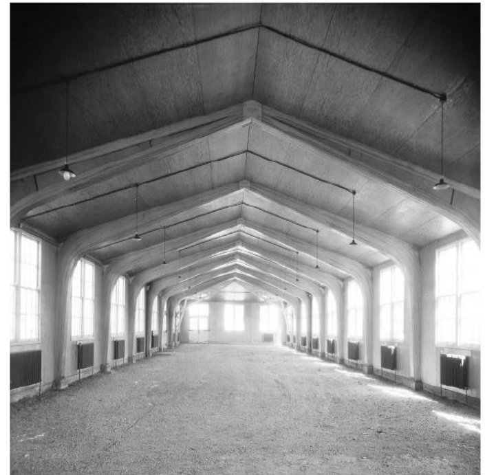
Figure 11-3. Erected in 1934 at the Forest Products Laboratory in Madison, Wisconsin, this building is one of the first constructed with glued-laminated timbers arched, designed, and built using engineering principles.
