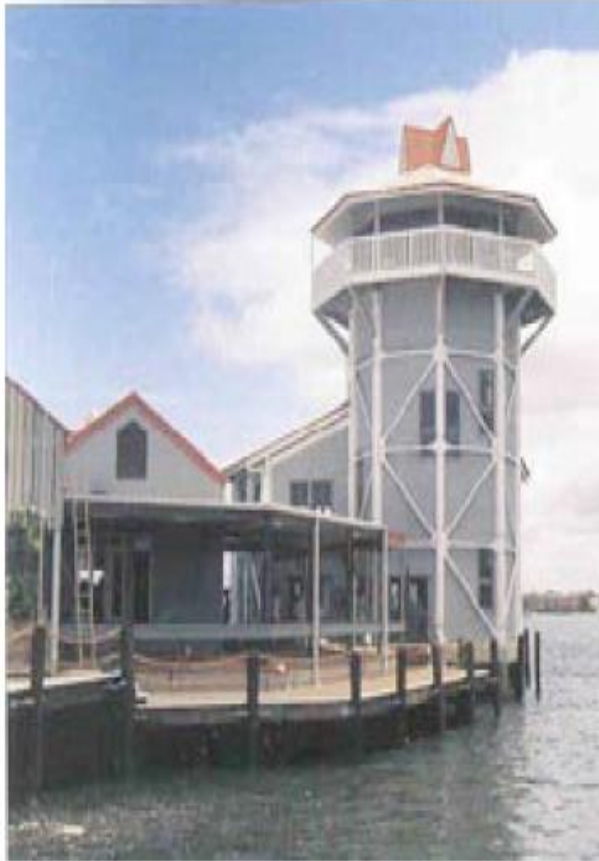
Buildings and wharf structures must be designed and protected against marine hazards.
